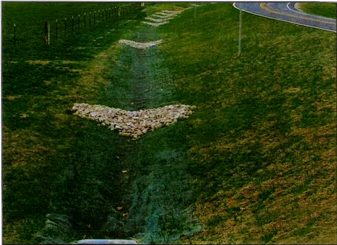
Figure 7 - Swale with Check Dams – ( https://megamanual.geosyntec.com/npsmanual/checkdams.aspx )
